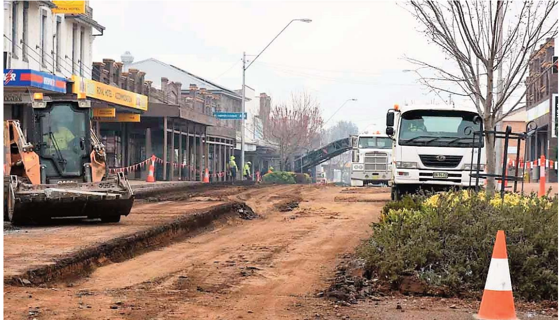
Bradley St is being dug up and will be realigned and resurfaced as part of Stage 2 of the CBD Upgrade
