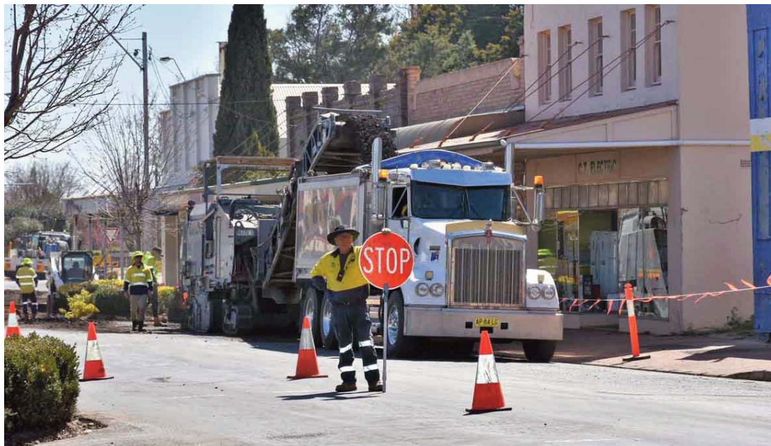
Work started on Monday and is expected to take two weeks
