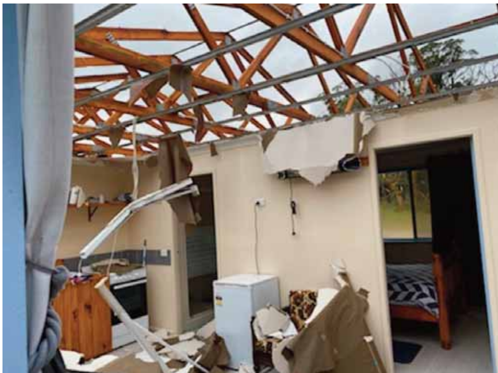
Ten buildings at Moredun Ponds were damaged in the storm including homes, sheds and farmstay cabins
