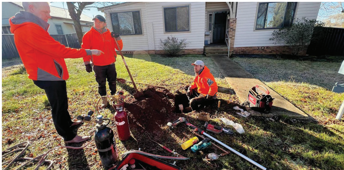
Council staff have installed approx. 800 water meters in Guyra
