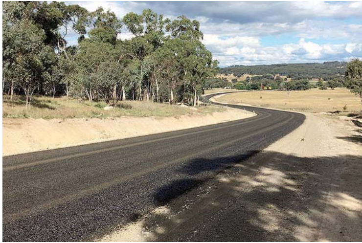
The newly sealed stretch of road
