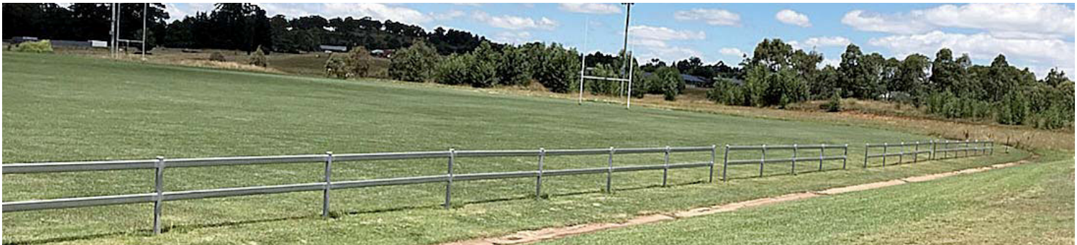
A dividing fence and a new PA system installed at the Guyra Sporting complex as a result of representations from Guyra Junior Rugby League
