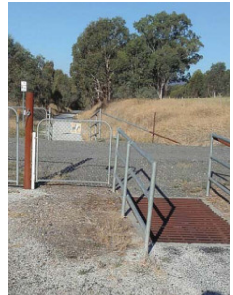
The High Country Rail Trail follows the old rail track with some unpaved, becoming paved as it nears civilisation. The paved trail is approximately 3 metres wide and when it passes through grazed areas ramps for bicycles, smaller gates for walkers and larger gates for stock movement were provided for safe access
