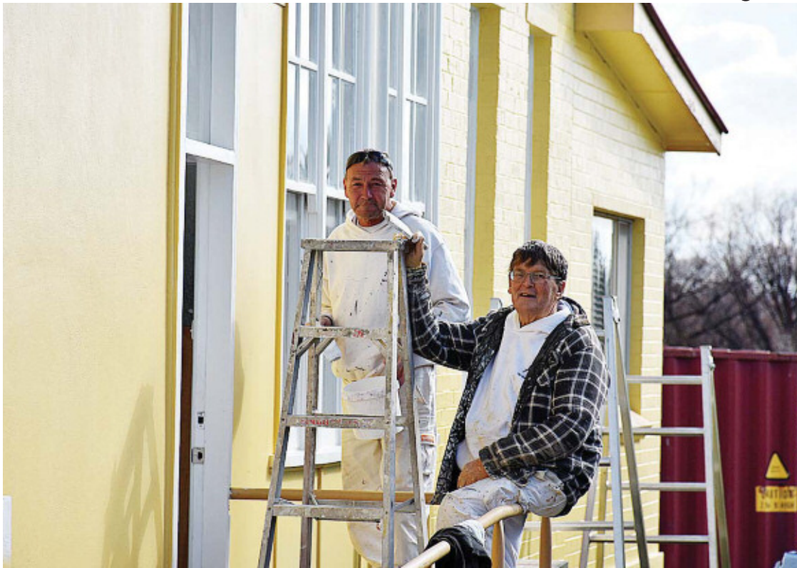
MUSEUM FACELIFT: Painters Quinn Larsen and Barry Cox at work on the outside of the building
