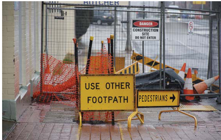
Council staff have removed barriers and temporarily repaired the footpath where one of the tanks is located. Work will now commence in February at the earliest
