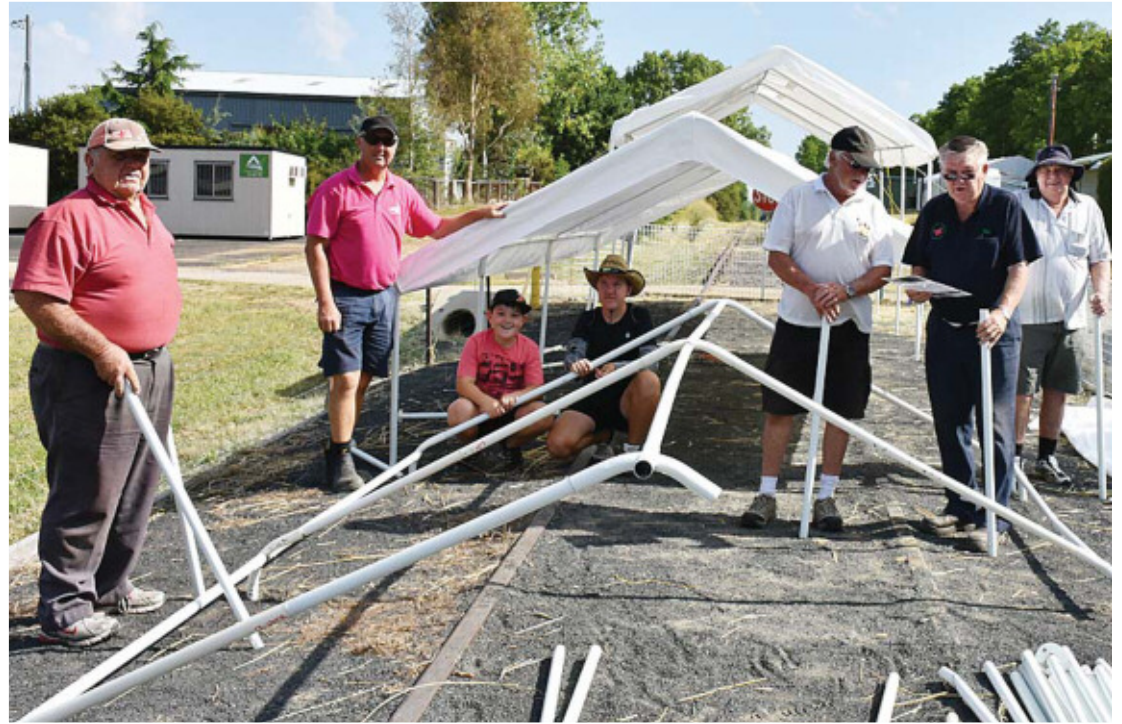
BACK ON TRACK: The Lamb and Potato Railway Station under construction Ron Lockyer Paul, Angus and Harris Dullaway, Peter Hansen, Sam Astle and Ray Martin
